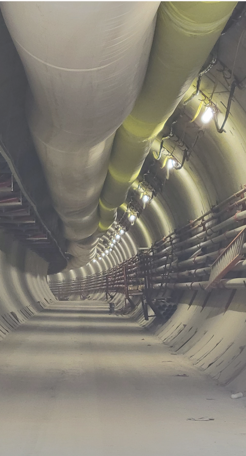
BROADWAY SUBWAY PROJECT, VANCOUVER · UNDERGROUND CROSSOVER TUNNELLING
